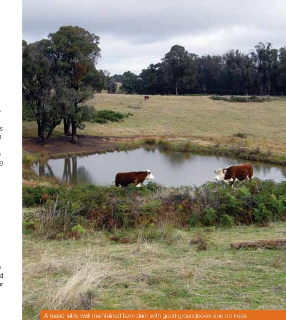
A reasonably well maintained farm dam with good groundcover and no trees on the dam wall. But there is some erosion occurring under the shade trees which are close to the dam. Fencing out eroding areas assists revegetation and improves water quality.
